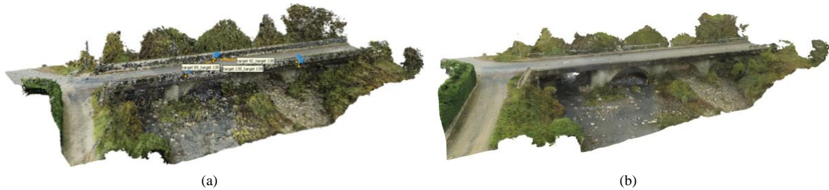
Figure 5 Geometrical survey of the Limentra bridge: (a) point cloud, (b) texturized tiled model.
