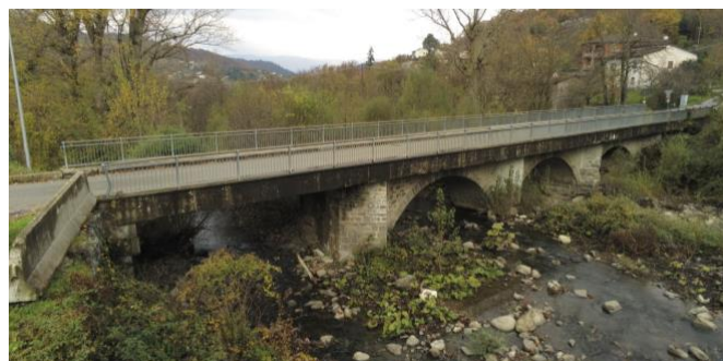
Figure 1 Overview of the Limentra bridge
