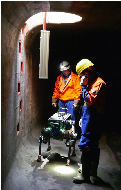
(a) ANYmal setup in the sewer
