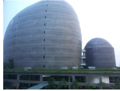
FIGURE 2. New Media Tower Building Multimedia Nusantara University
