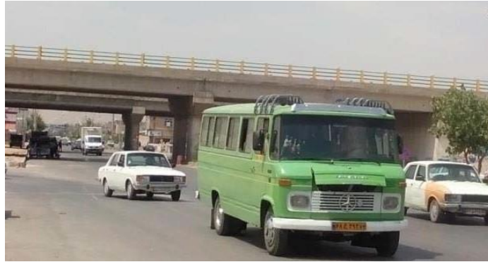
Figure 6 View of Mianrood Bridge and its crater on the Belt Road
