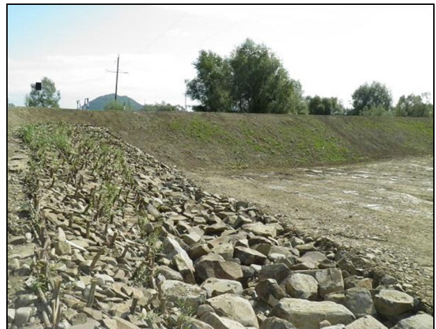
Fig. 7. Reconstructed protective dam to protect the city of Khust from floods (2011) [21].
