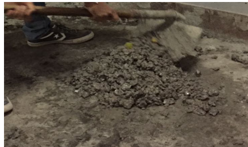
Figure 5 Mixing of Geopolymer concrete
