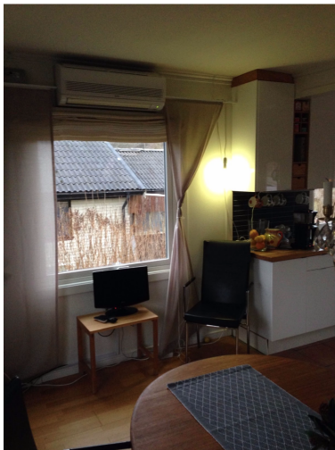
Figure 2: First prototype near the kitchen in the dining room
